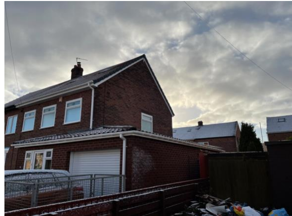
Figure 9: B1 - gable end/garage.
