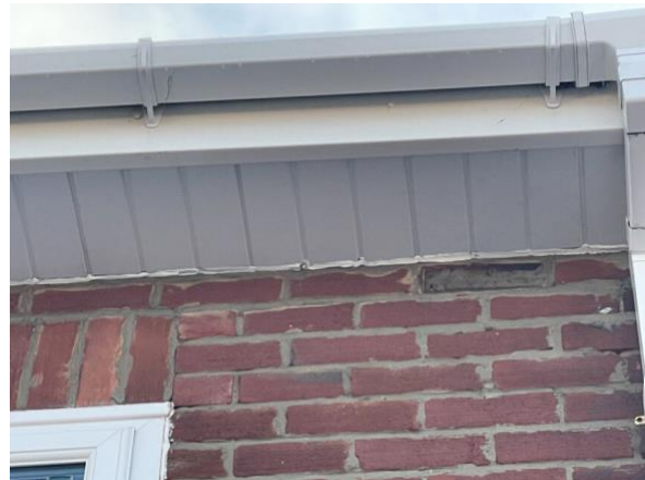
Figure 11: B1 - soffit box of the main house.
